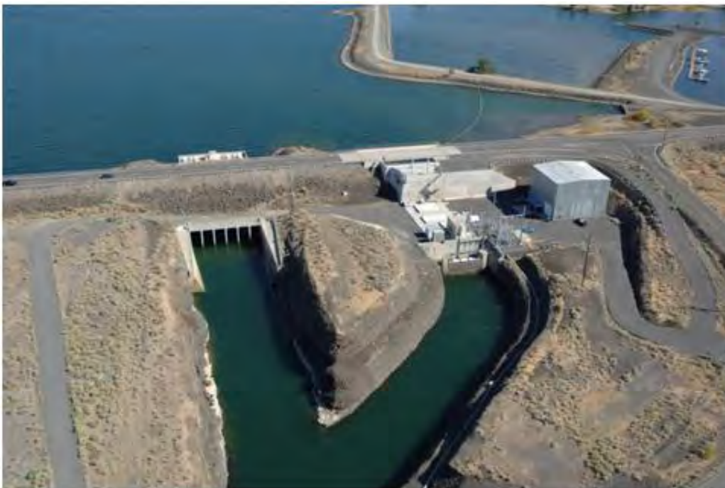
Photograph 2-4. Main Canal Headworks and Powerplant at Dry Falls Dam.
