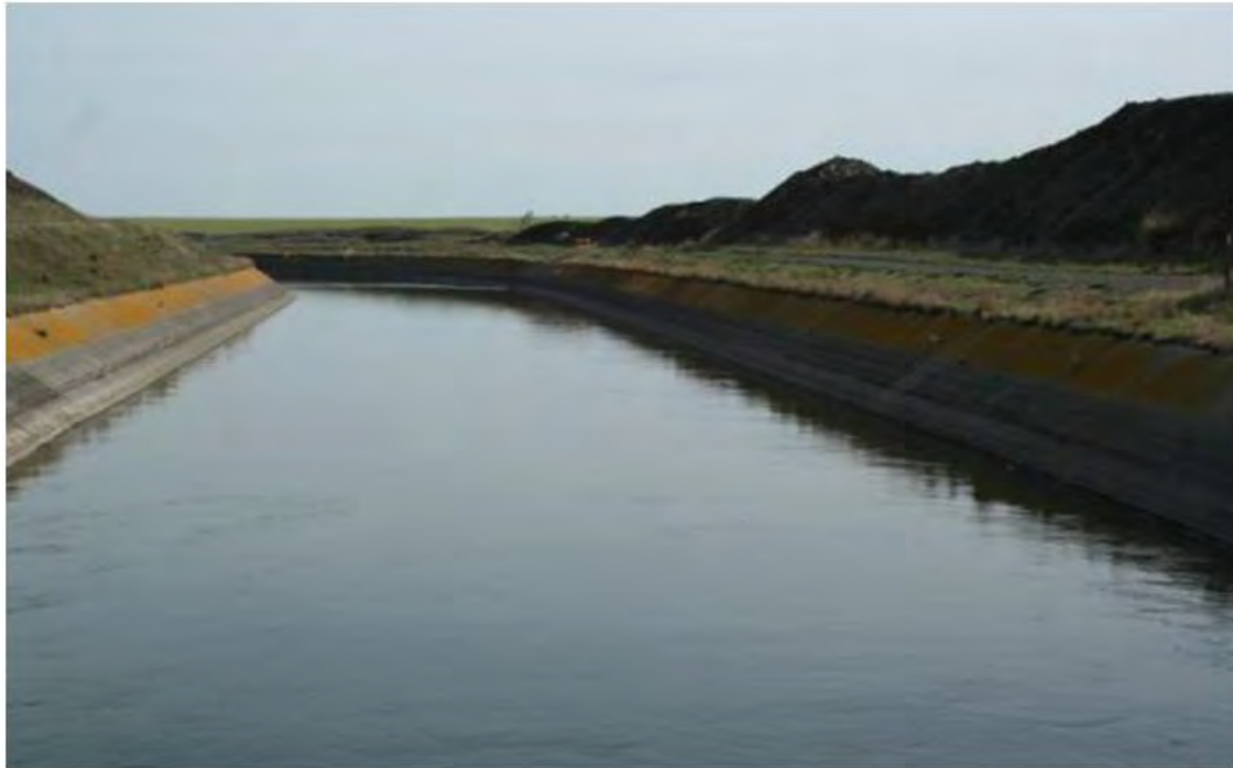
Photograph 3-1. CBP Main Canal.
