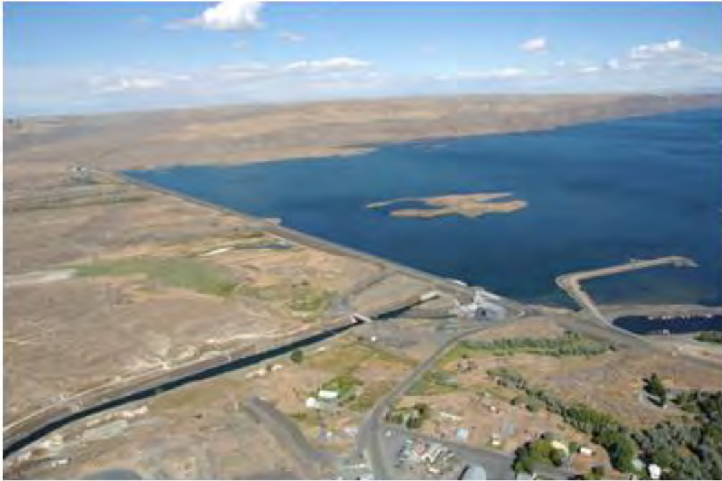
Photograph 2-3. Banks Lake, Dry Falls Dam, and the Main Canal.
